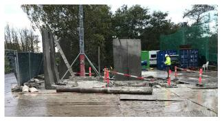
Fig. 11: Protection from UXOs when performing HDD drillings in an old military shooting range.
