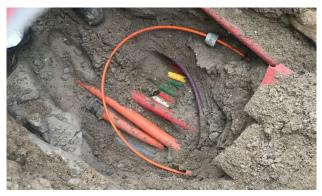
Fig. 12: Digging a hole is not so simple in an urban environment where a lot of different distribution lines are fighting over the same corridors.
