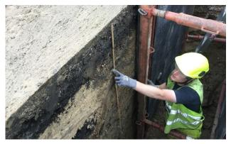
Fig. 13: At certain places it might be necessary to install the cables very deep, in order to ensure clearance distances to other infrastructure.
